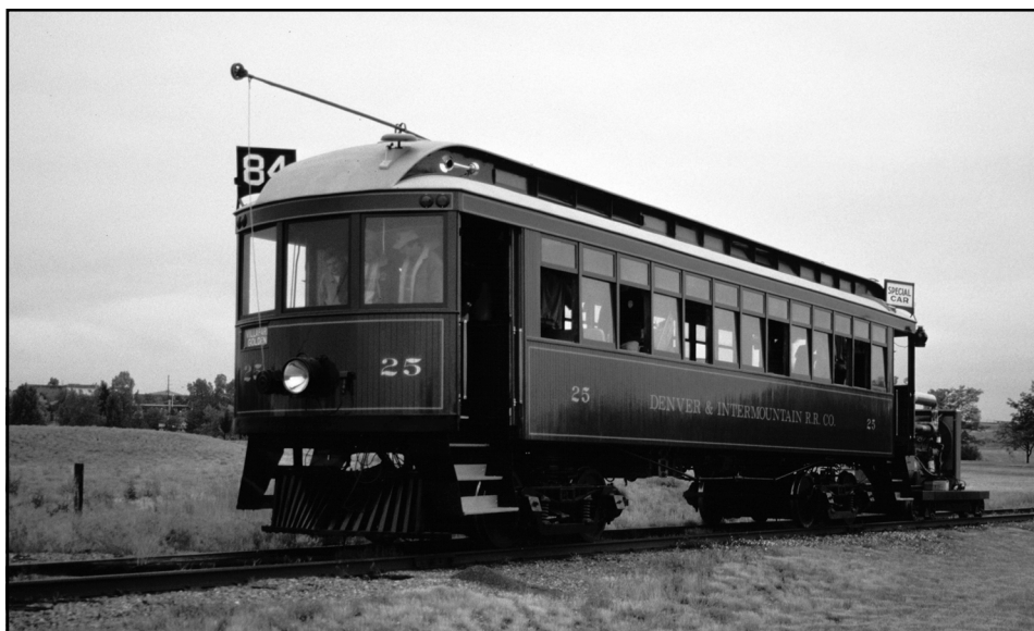
Car No. 25 followed by the Diesel generator during the 6/26/00 test run at the Denver Federal Center. – Photo © Steve Mason
